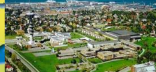
Marine Technology Centre, Trondheim
